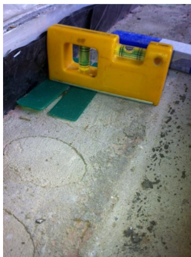
Photo 1 Levelling & packing front to back
