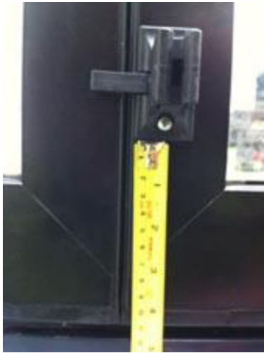
Photo 13 Female panel catch section with arm projecting across adjacent panel
