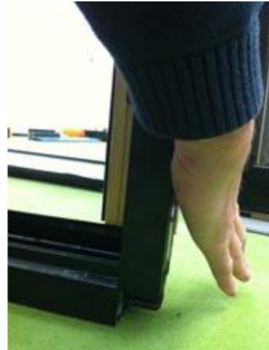
Photo 7 Use the palm of your hand to slide the jambs into the tracks
