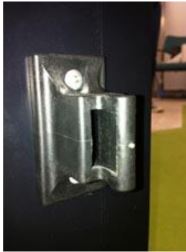
Photo 14 Male panel catch section with cut-out which should face the opposite way of the projecting arm of the female section
