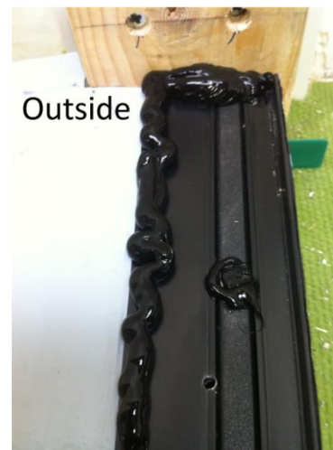
Photo 8 Silicone bead between sill and track
