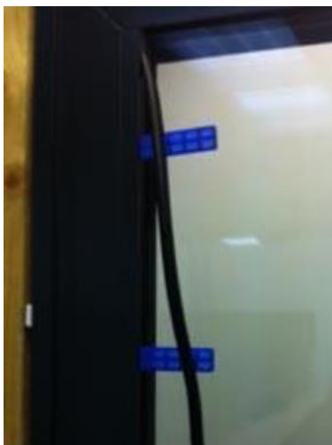
Photo 6 Insert packers to secure bead and facilitate gasket insertion.
