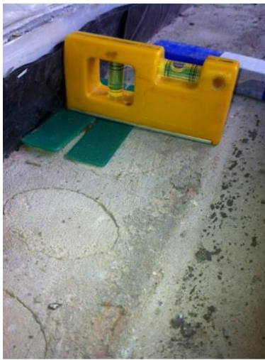
Photo 1 Levelling & packing front to back
