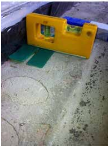
Photo 1 Levelling & packing front to back
