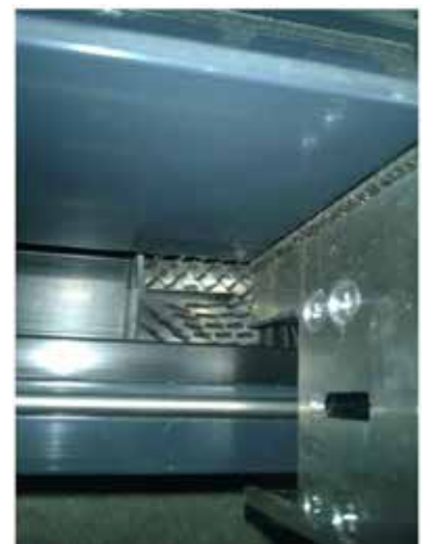
Photo 7 Please note the bottom brush block must be sealed into the track with silicone to prevent water passing beside the block
