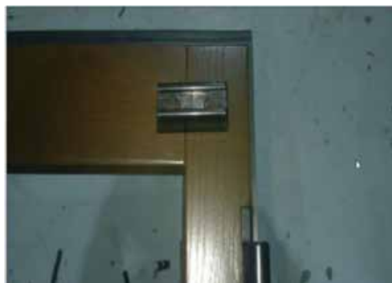
Photo 16 Panel catch fitted horizontally on panel
