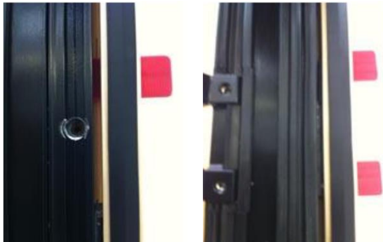
Photo 5 Pre-drilled fixing location
