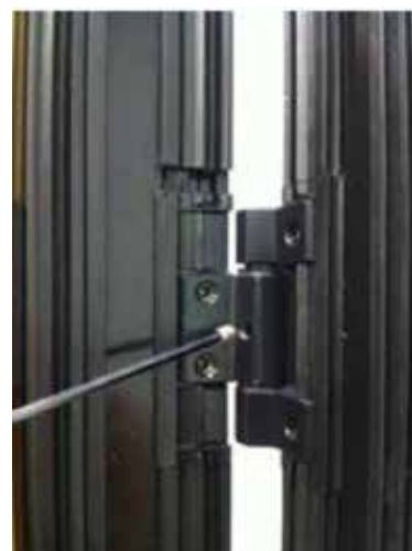
Photo 11 Securing hinge pins
