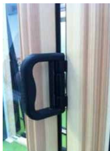
Photo 9 Fitted pull handle to outward opening systems
