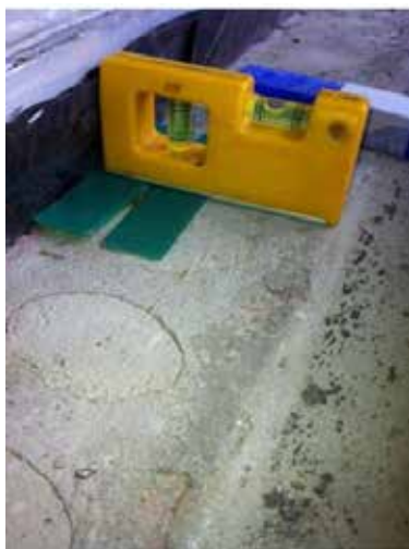
Photo 1 Levelling & packing front to back
