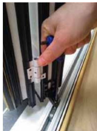
Photo 10 Adjusting the setup height
