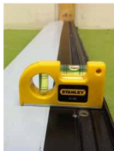
Photo 4 Checking sill is level
