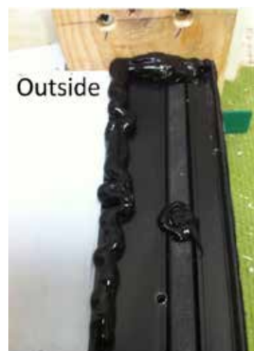
Photo 8 Silicone bead between sill and track
