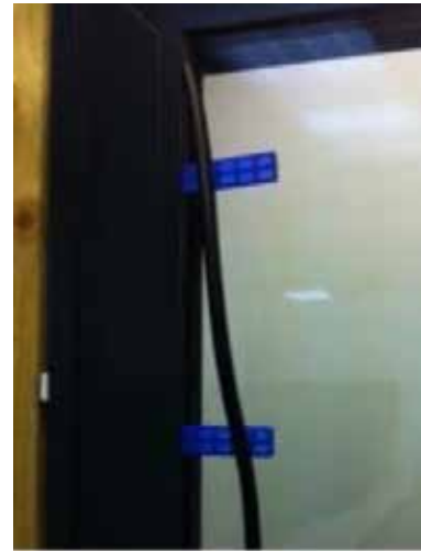
Photo 16 Insert packers to secure bead and facilitate gasket insertion.
