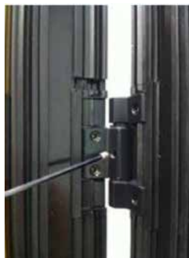
Photo 12 Securing hinge pins
