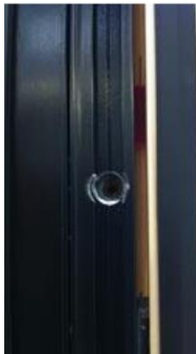
Photo 5 Pre-drilled fixing location
