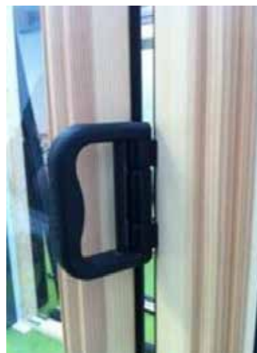
Photo 11 Fitted pull handle to outward opening systems
