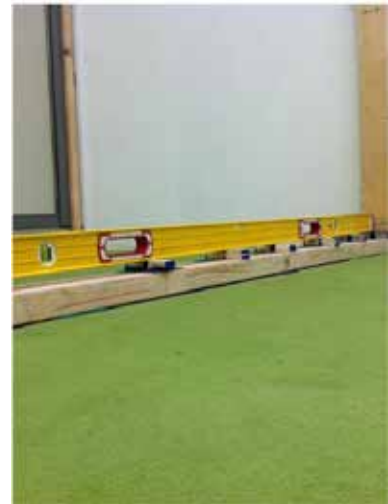
Photo 3 Levelling left to right
