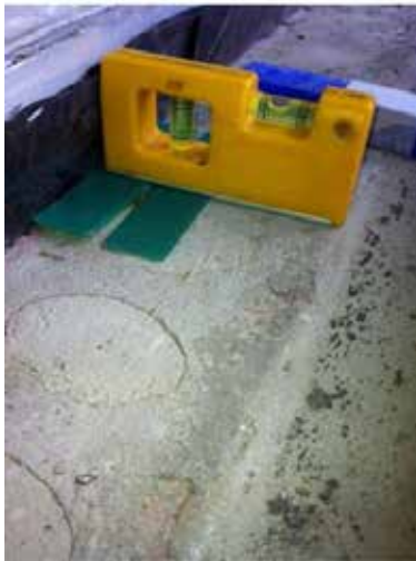
Photo 1 Levelling & packing front to back
