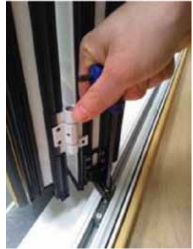
Photo 10 Adjusting the setup height
