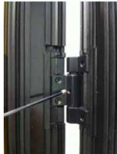
Photo 11 Securing hinge pins
