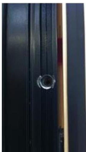
Photo 5 Pre-drilled fixing location
