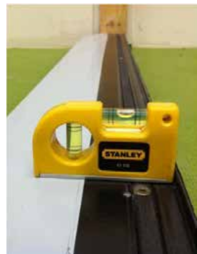
Photo 4 Checking sill is level
