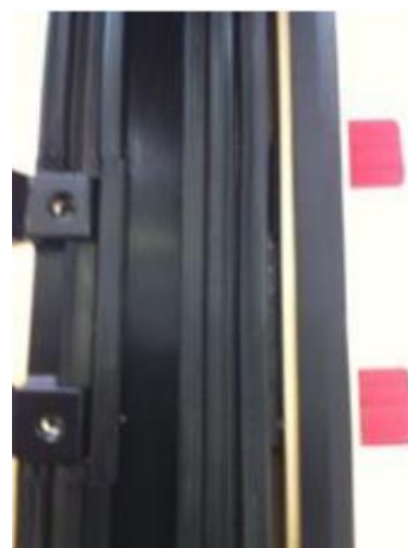
Photo 6 Gasket covers pre-drilled fixing location and screw once fitted
