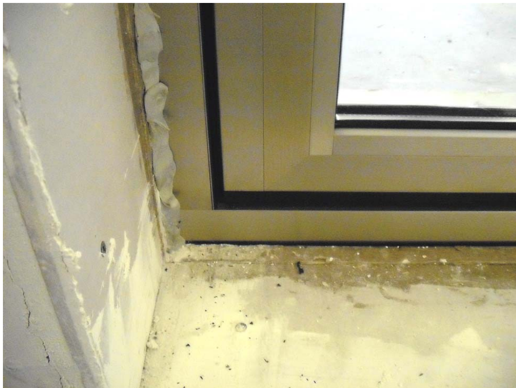
Fig. 4: View Receiving Room, Detail connection floor
