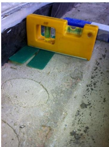
Photo 1 Levelling & packing front to back
