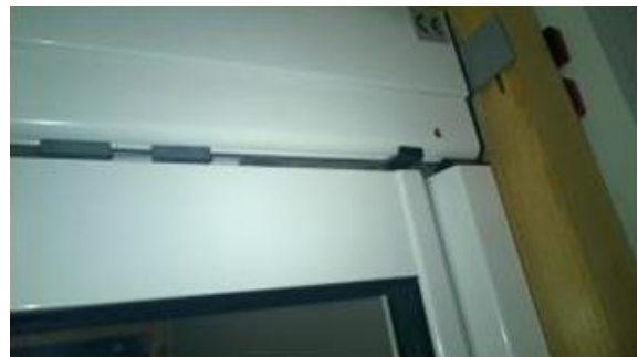
Photo 13 Lead panel pushed up to side jamb, Locking lever now has to be turned 90° away from the side jamb
