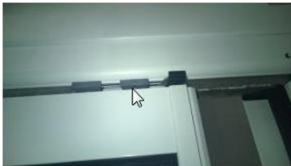
Photo 12 Locking lever turned 180° to cut-out side of top track.
