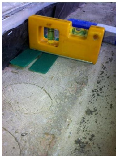
Photo 1 Levelling & packing front to back
