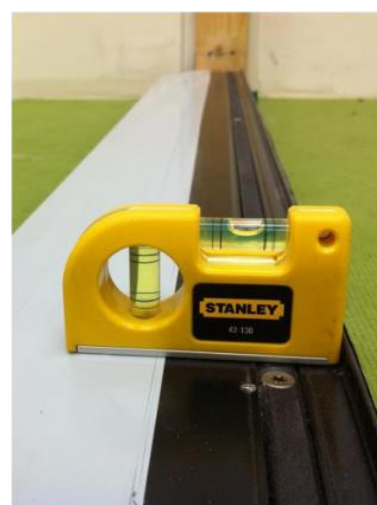
Photo 4 Checking sill is level
