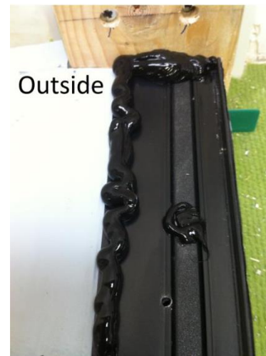
Photo 8 Silicone bead between sill and track
