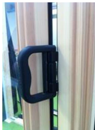
Photo 11 Fitted pull handle to outward opening systems
