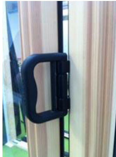
Photo 11 Fitted pull handle to outward opening systems
