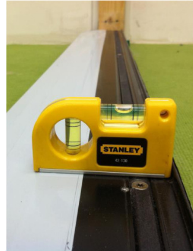
Photo 4 Checking sill is level
