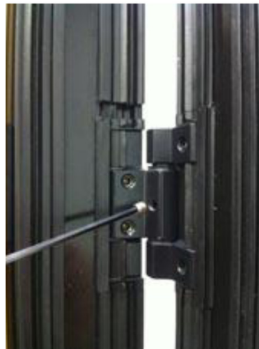
Photo 12 Securing hinge pins
