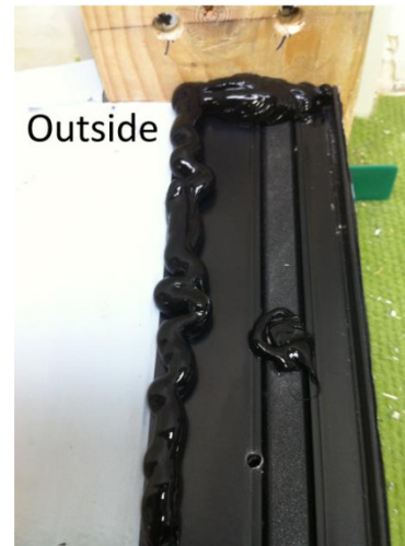
Photo 8 Silicone bead between sill and track
