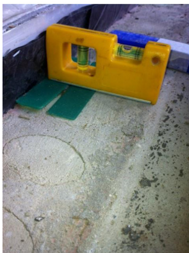
Photo 1 Levelling & packing front to back
