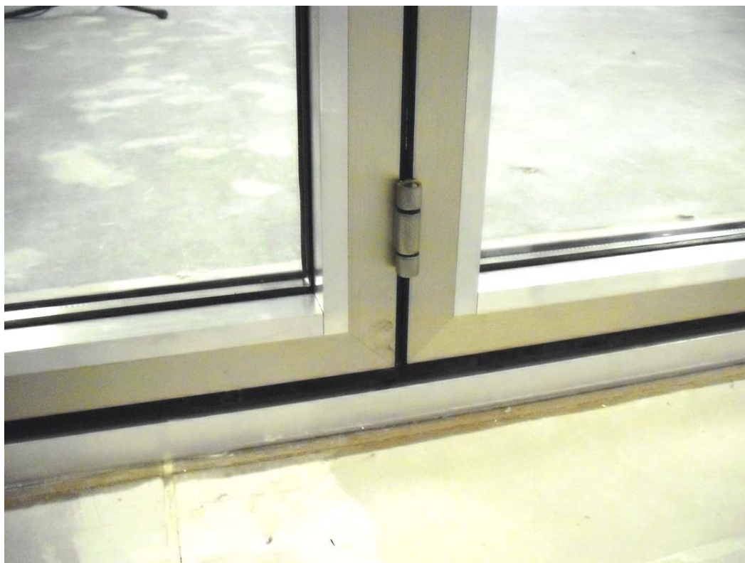
Fig. 4: View Receiving Room, Detail connection floor
