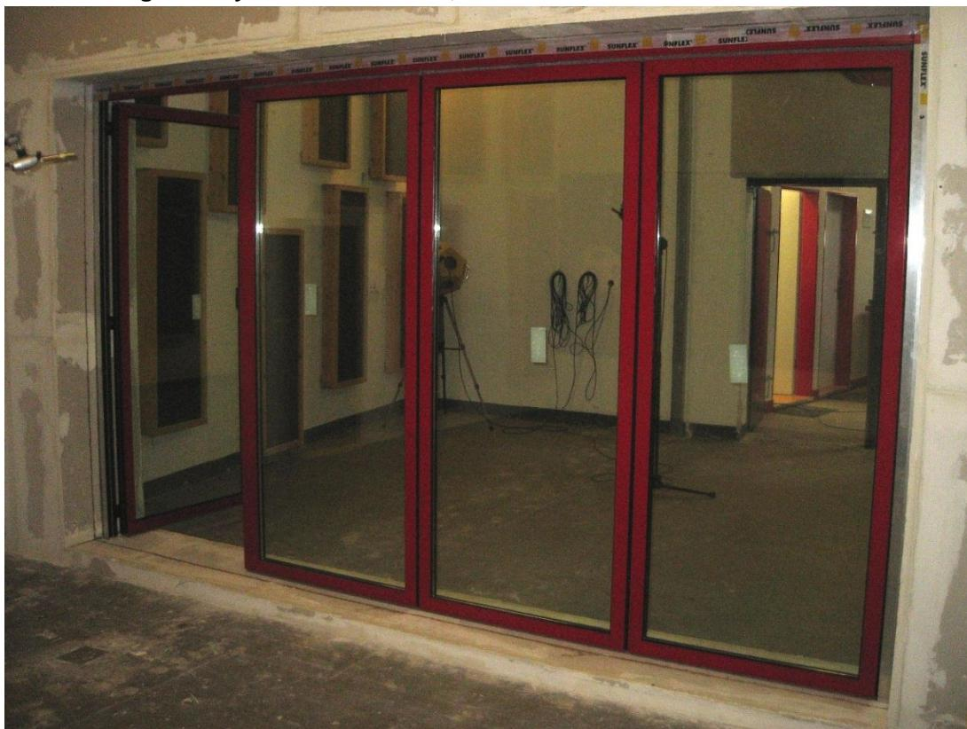
Fig. 2: Horizontal-Sliding-Wall-System SF 50 H-S-W, View Transmission Room, Detail connection ceiling
