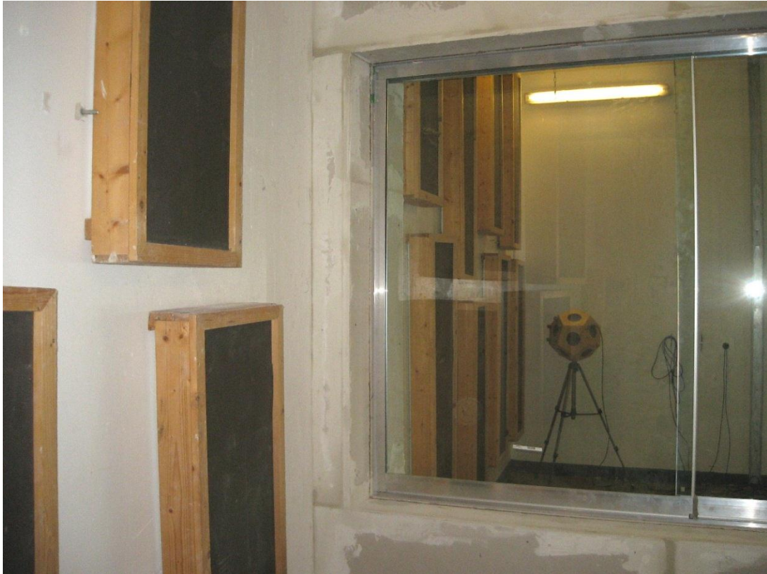
Fig. 1: All-Glass Sliding System SF 20, Partial View Transmission Room
