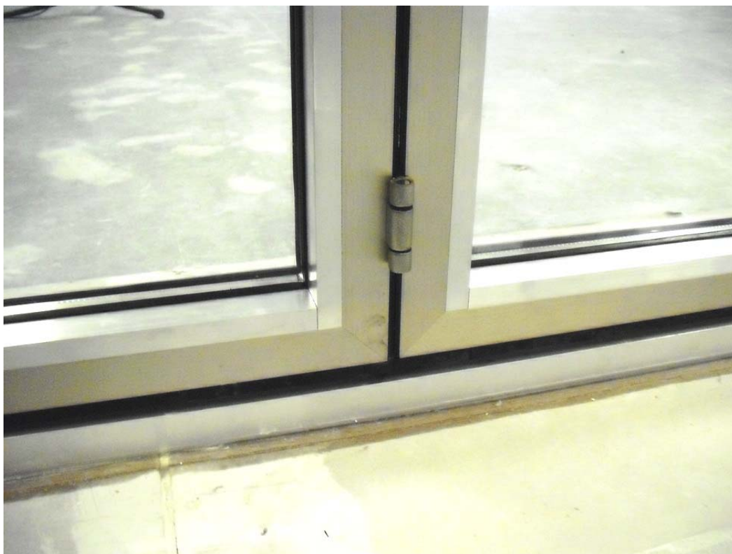
Fig. 4: View Receiving Room, Detail connection floor
