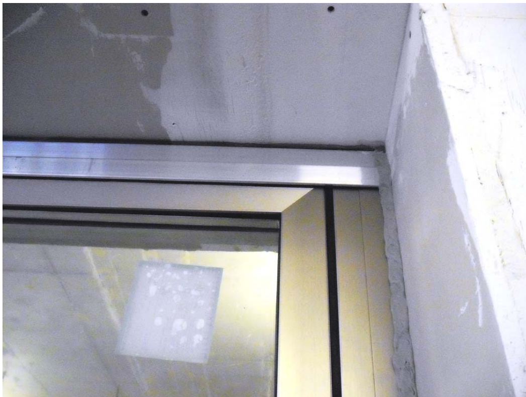
Fig. 2: View Transmission Room, Detail connection ceiling
