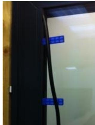
*Photo 15 – insert packers to secure bead and facilitate gasket insertion.*
