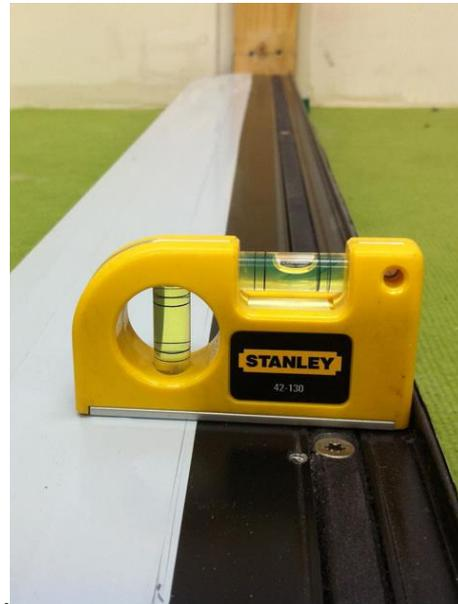
*Photo 4 Checking sill is level*
