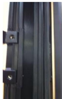
*Photo 6 --Gasket covers pre-drilled fixing location and screw once fitted*
