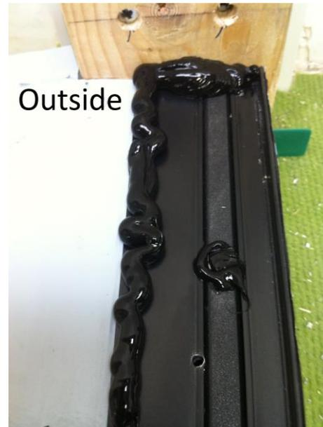
Photo 8 – Silicone bead between sill and track
