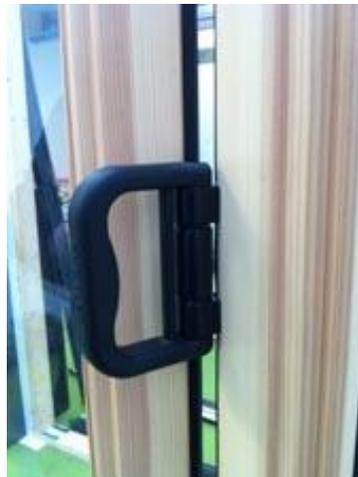
*Photo 9 – fitted pull handle to outward opening systems*
