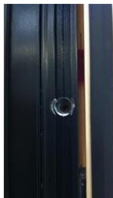
*Photo 5 - Pre-drilled fixing location*
