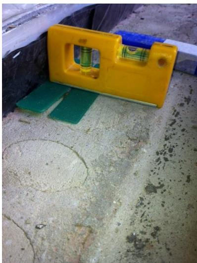
*Photo 1: Levelling & packing front to back*
