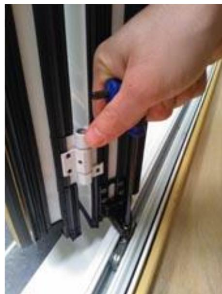
*Photo 10 – Adjusting the setup height*
