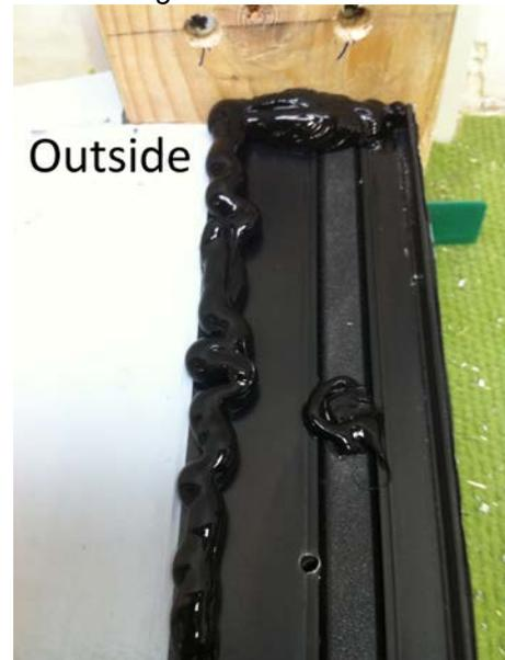
*Photo 5 – Silicone bead between sill and track*
